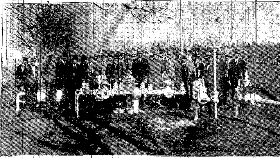
Mayor W. M. Orr turned the valve which marks completion of a system bringing the new fuel to Wayne for distribution. Dr. J. G. W. Lewis addressed gas company and city officials and others briefly after the valve was opened. The People's Gas company was host to 20 men at noon luncheon in Hotel Stratton afterward.
